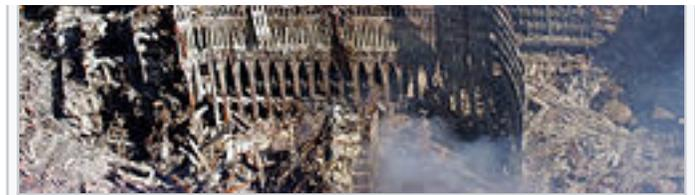
Portions of the outer shell of the North Tower lean against the remains of 6 WTC which suffered massive damage when the North Tower collapsed. The remains of 7 WTC are at upper right
