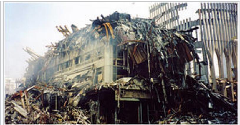
The outer shell of the South Tower (tower 2) of the WTC is still standing at right. The 22-story [Marriott Hotel](#) in the foreground was crushed when the south tower collapsed.
