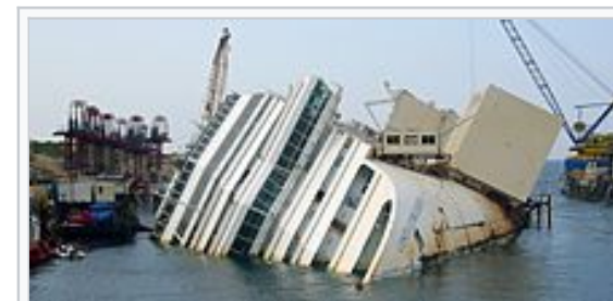
Costa Concordia salvage operation in progress ↗
